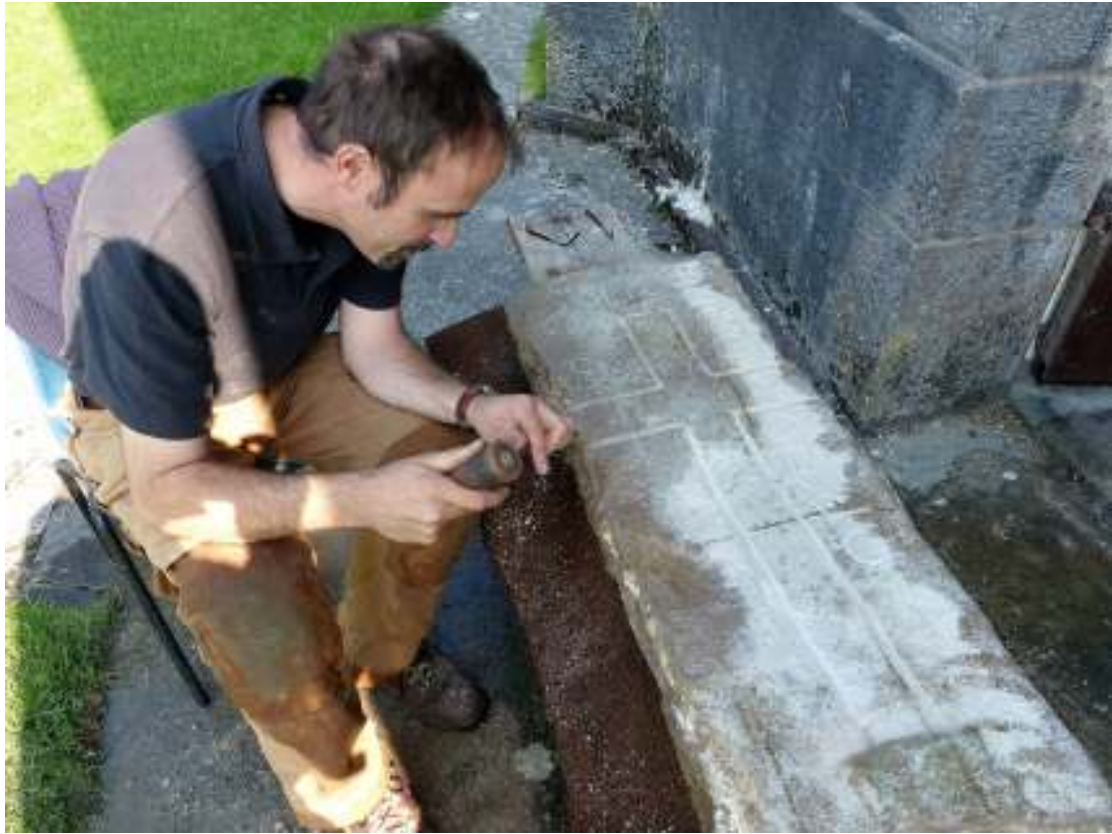
Fig. 4; After extraction from the wall: removal by hand of attached cement mortar from sides and rear of carving.
