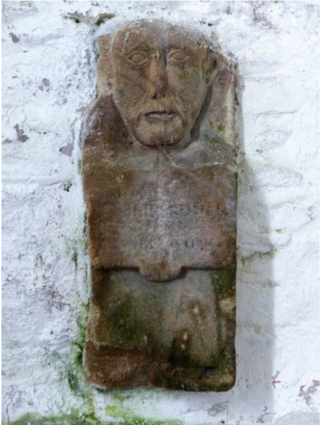
Fig. 2; One of the pieces prior to works, showing harmful biological growth and efflorescence on the stone surface due to serious dampness in the wall.
